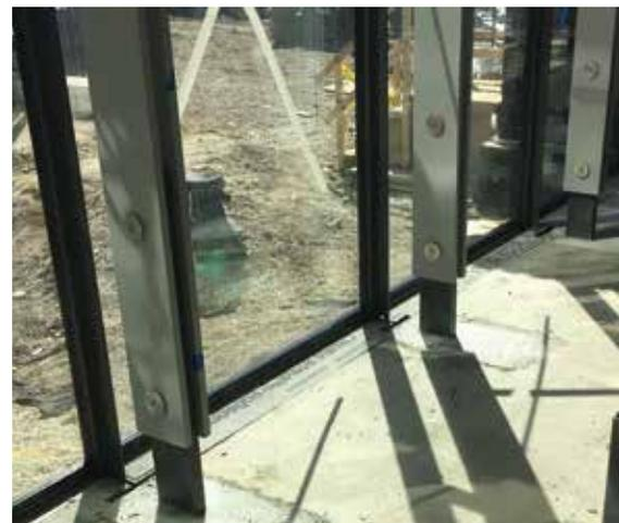
View of the erected steel paired plate mullions and two-bolt connection at the base of the glass wall.
