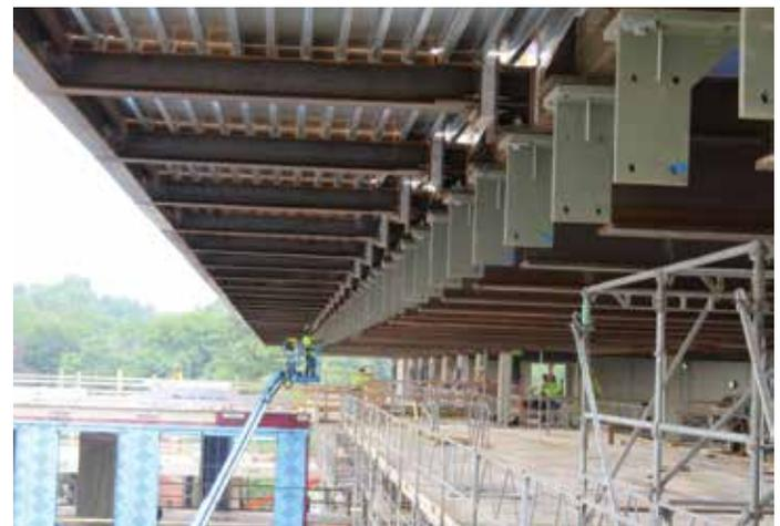
View of the erected roof framing and curtain wall connection plates at the top of the wall.
