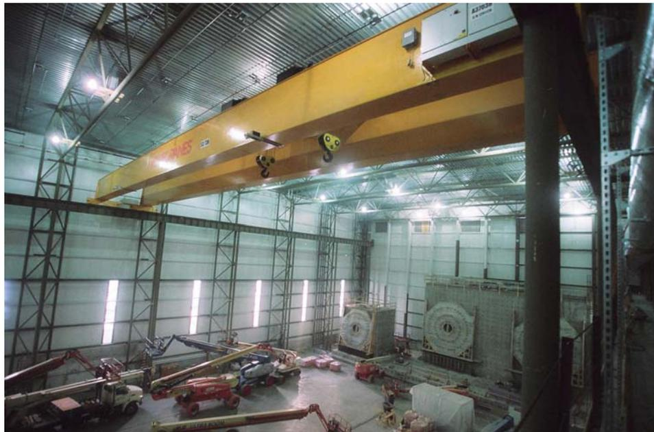
**Figure 12. Crane girders and runway beams, looking southwest.**
