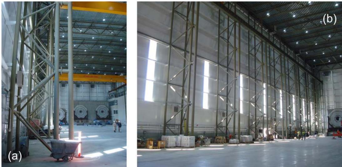
**Figure 6. (a) South trussed frames and crane columns facing west. (b) South trussed frames, crane columns, midheight drag elements, and runway beam facing southwest.**
